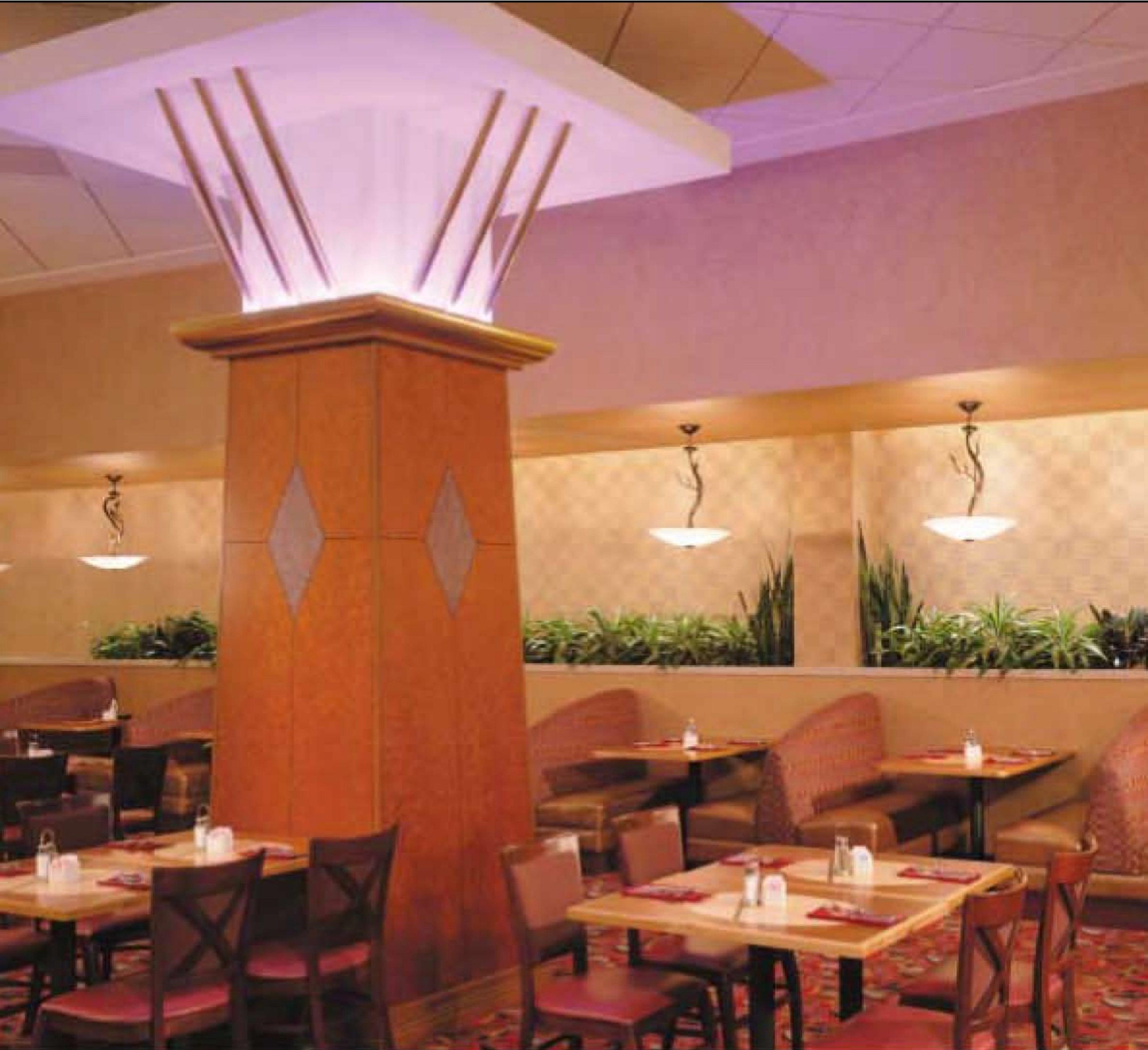
THE DRAMATIC CHERRY COLUMNS were pre-manufactured by the AWI member firm. Column tops are made from a series of aluminum extrusions finished in brass.
